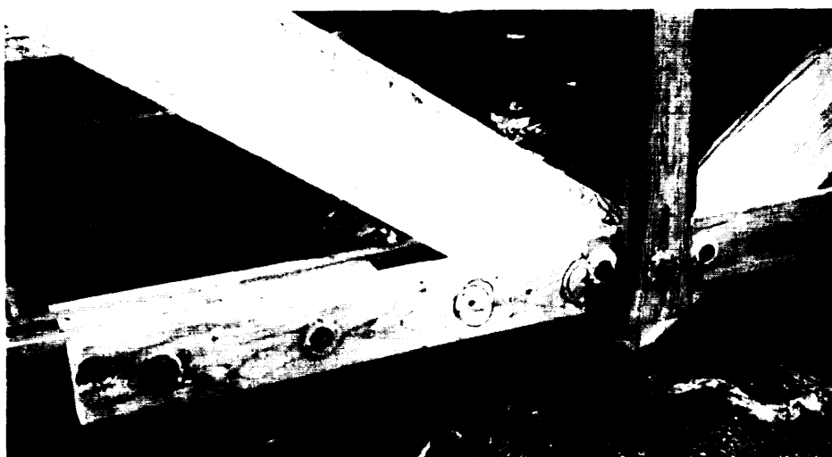
(B) OLD SPLICE PLATE REMOVED AND LONGER SPLICE PLATE ADDED
